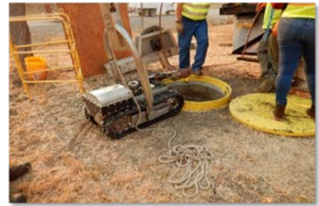
Multi-Sensor Inspection (dry pipe)
