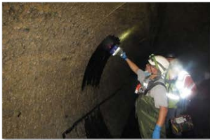
Confined Space Inspection
