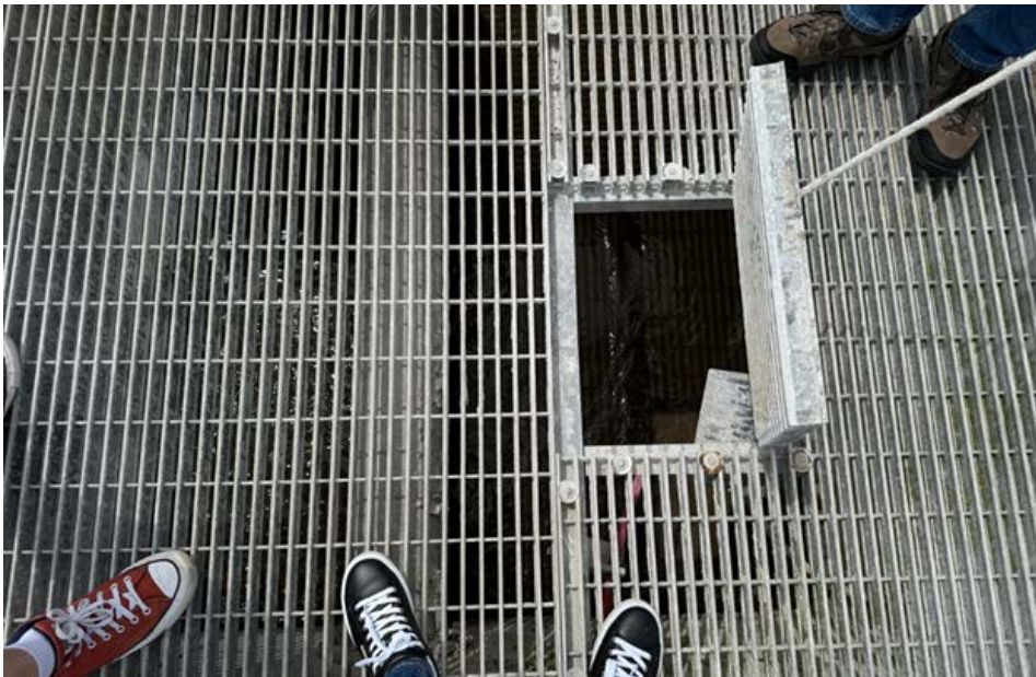
Logansport Utilities Wastewater Treatment Plant
