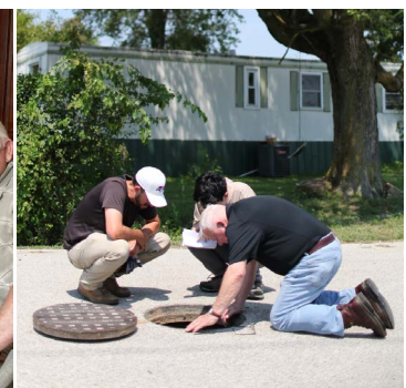
Flow meter location survey in the Switz City wastewater system
