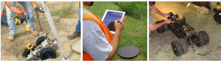
Fig. 6. Robust CCTV Crawler System Deployment Into the NSPPI
