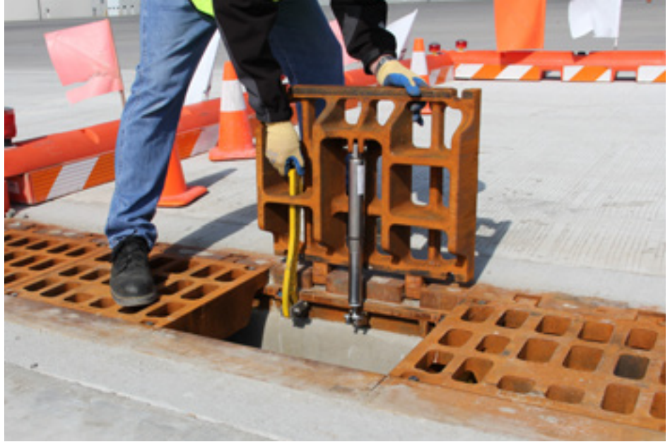
Self-engaging safety bar with optional mechanical lift assist make the hinged trench covers and grates safe and easy to use.
