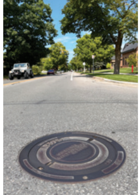
9 years after installation (August 28, 2023)
