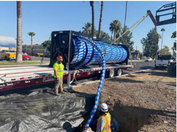
FFRPP can be pulled 2000 to 8000 feet between pits
