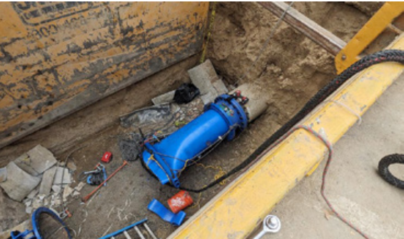
Installation requires only two small access pits
