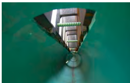
View inside PVC pipe
