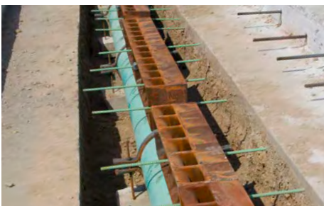
Linear slotted drain vane grate during installation
