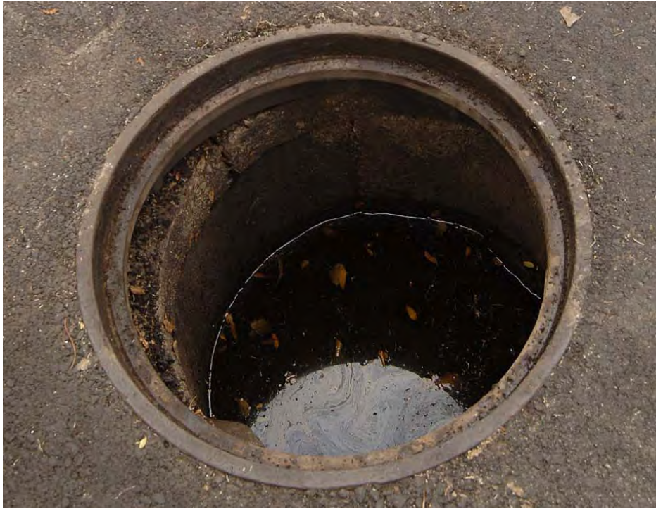
Missing and stolen covers are dangerous to pedestrians and motorists. Make sure they are properly secured against the hazards in their environment.
