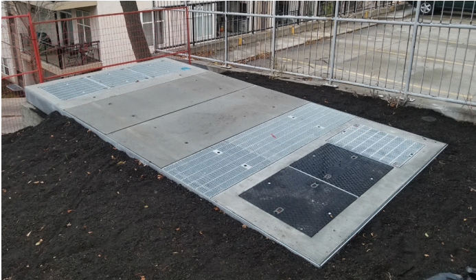
This hybrid assembly installed on a power vault in Alberta, Canada combines steel grating and composite rectangle panels along with a concrete infill frame.
