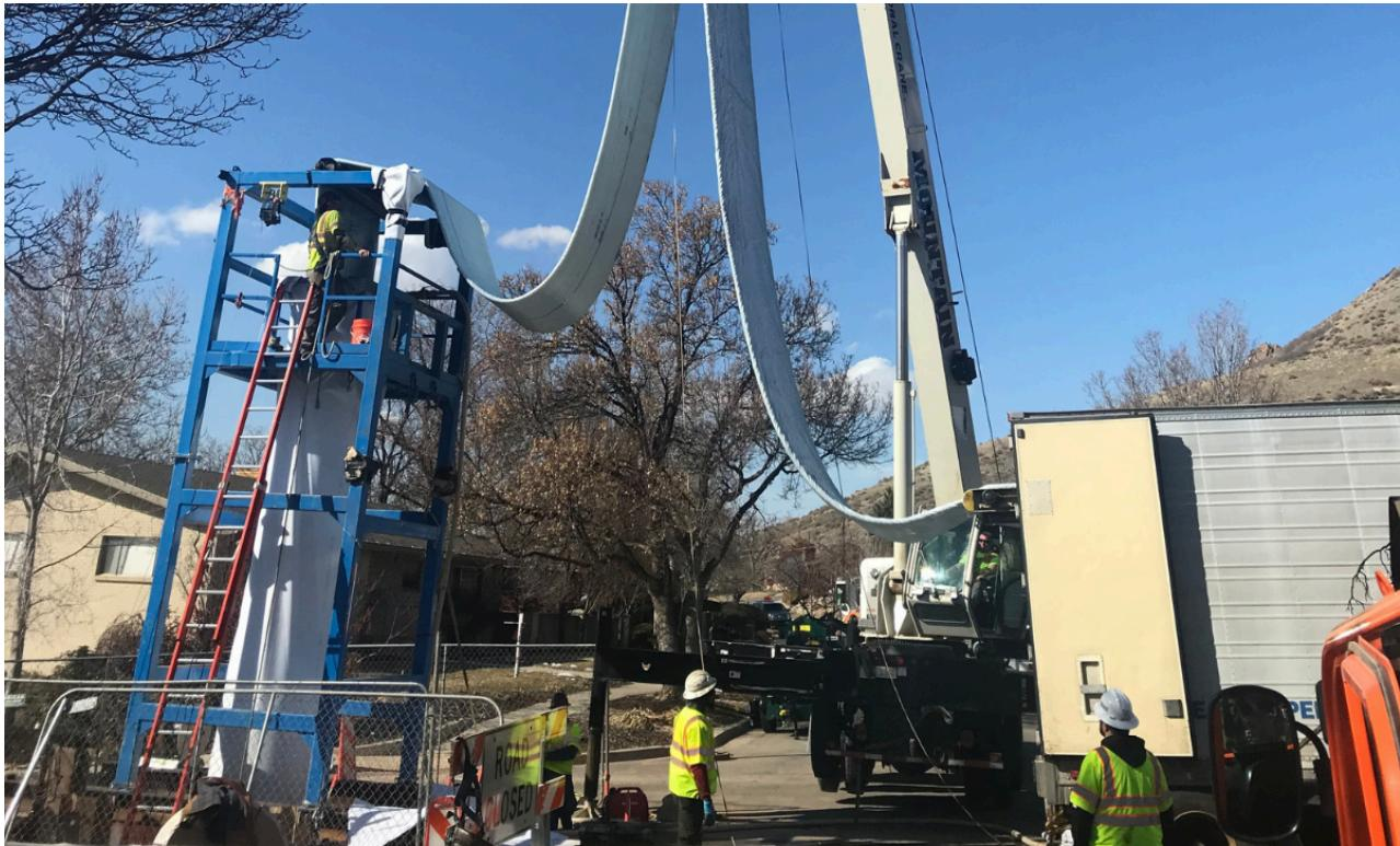
The Upper Conduit in Salt Lake City is a critical water transmission pipeline constructed utilising various types of concrete pipes, including prestressed concrete cylinder pipe (PCCP), reinforced concrete cylinder pipe (RCCP) and steel cylinder concrete pipe (SCCP).
