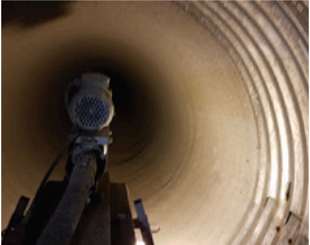
Centrifugal casting of GeoSpray mortar.
