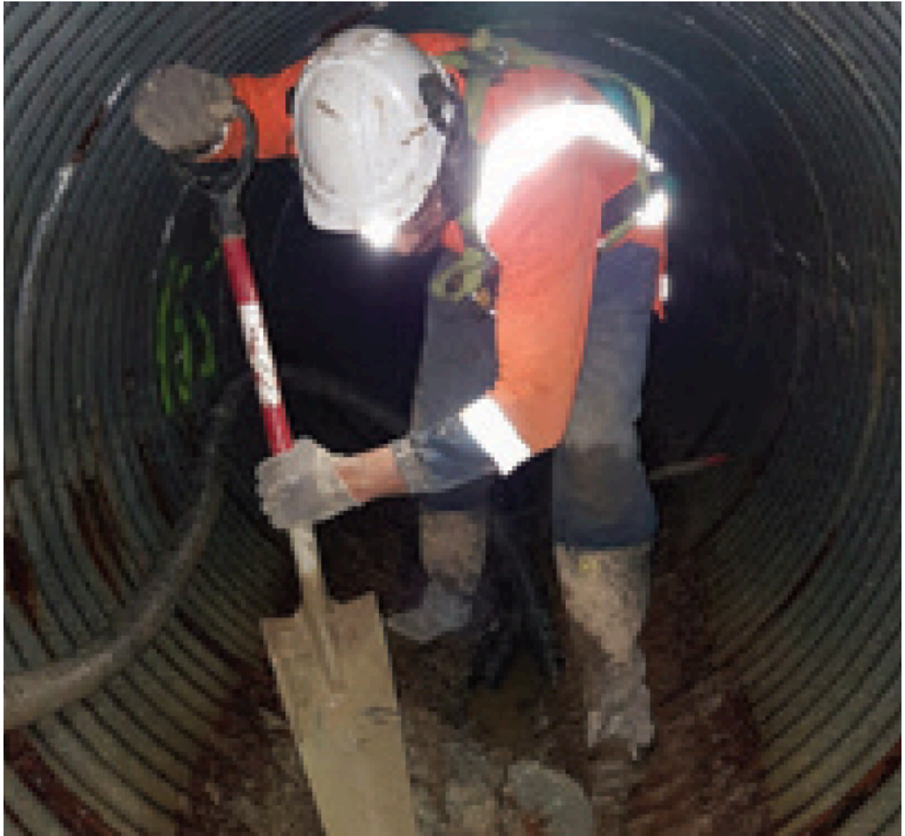
Excavation of debris within the culvert invert
