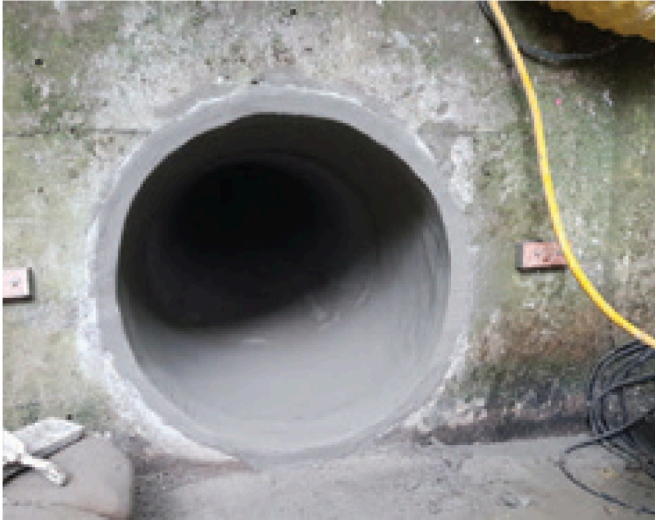
Completed lining with GeoSpray mortar at inlet.
