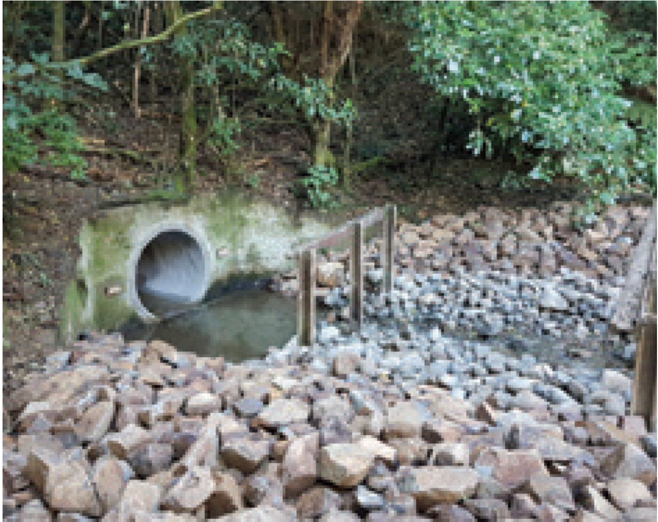
Completed culvert with GeoSpray mortar and riprap surrounding exterior.
