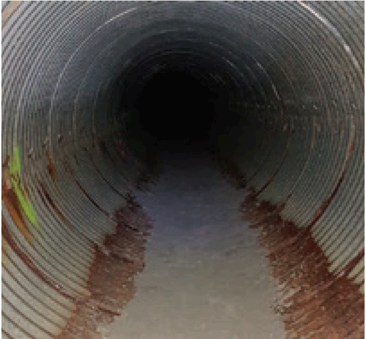
Invert repaired and ready for GeoSpray mortar casting.
