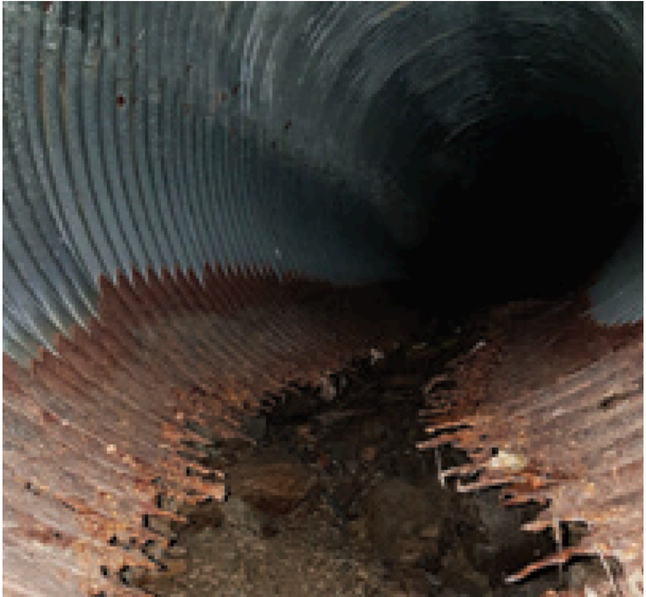
Condition of invert prior to GeoSpray coating.
