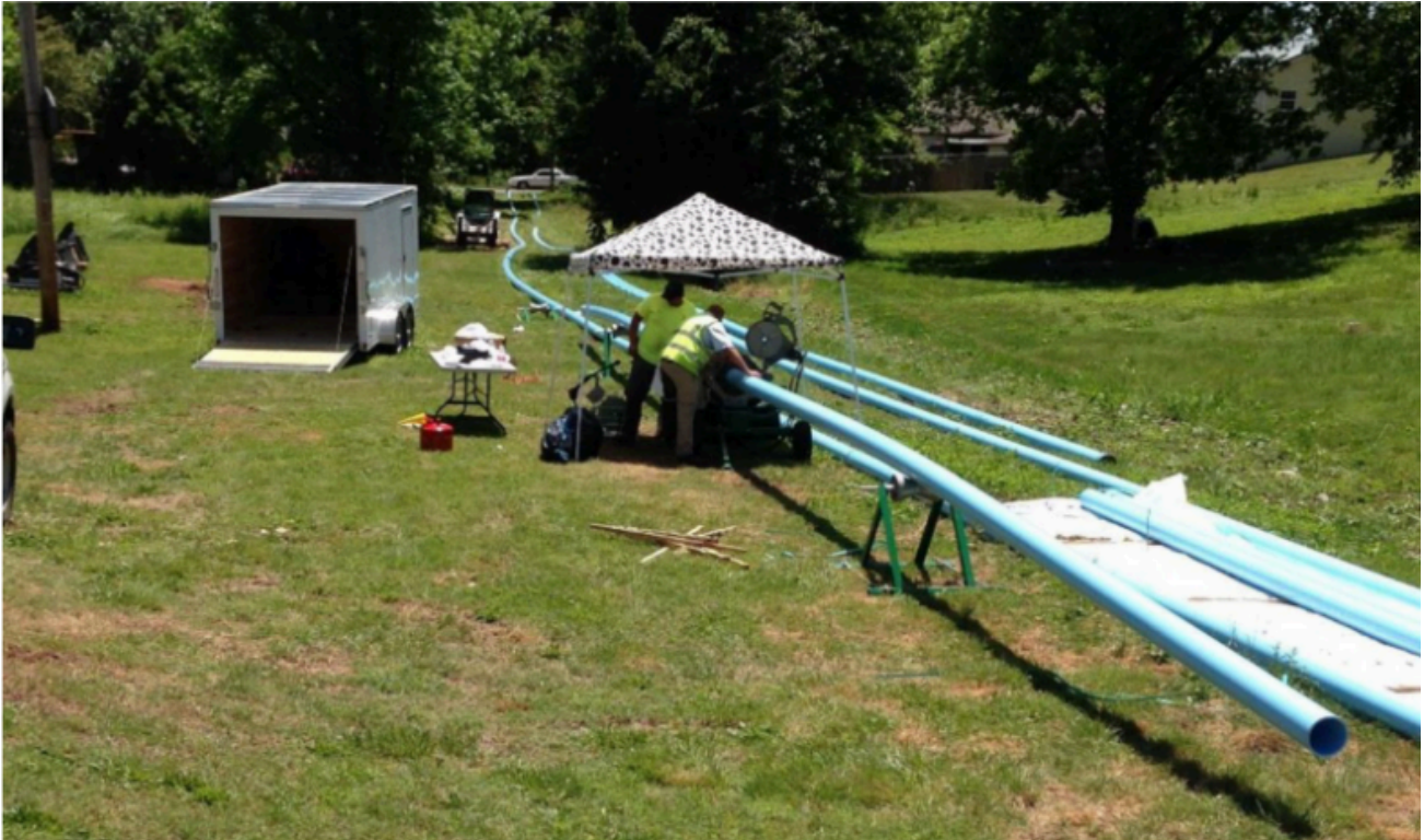
Fusion of several lengths of Fusible PVC® pipe for installation
