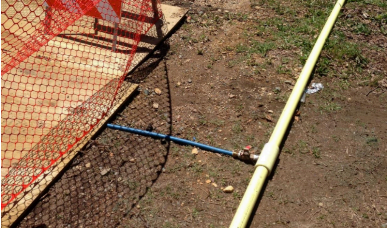
Temporary water service connection
