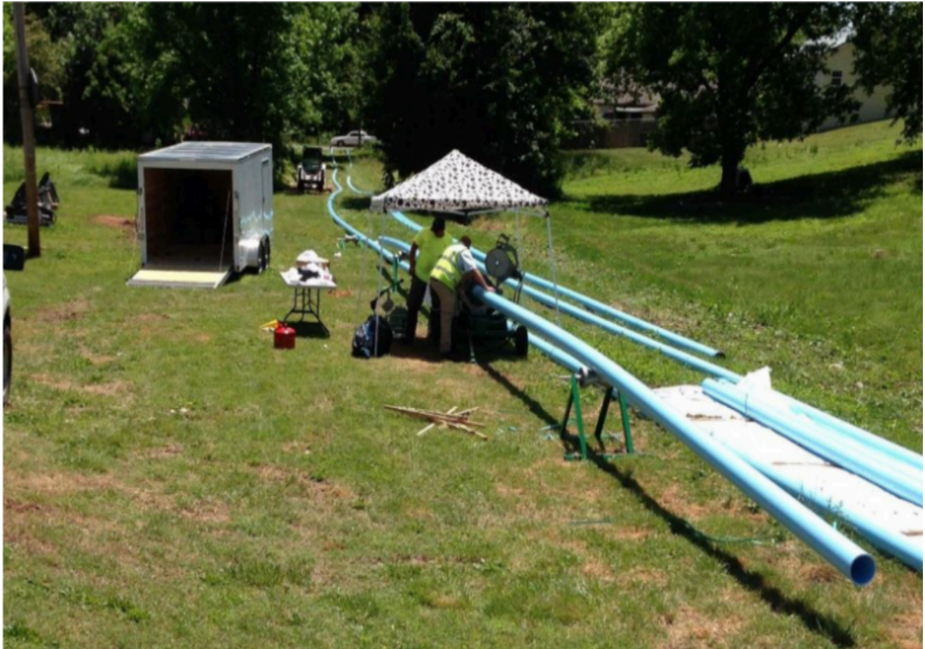
Fusion of several lengths of Fusible PVC® pipe for installation
