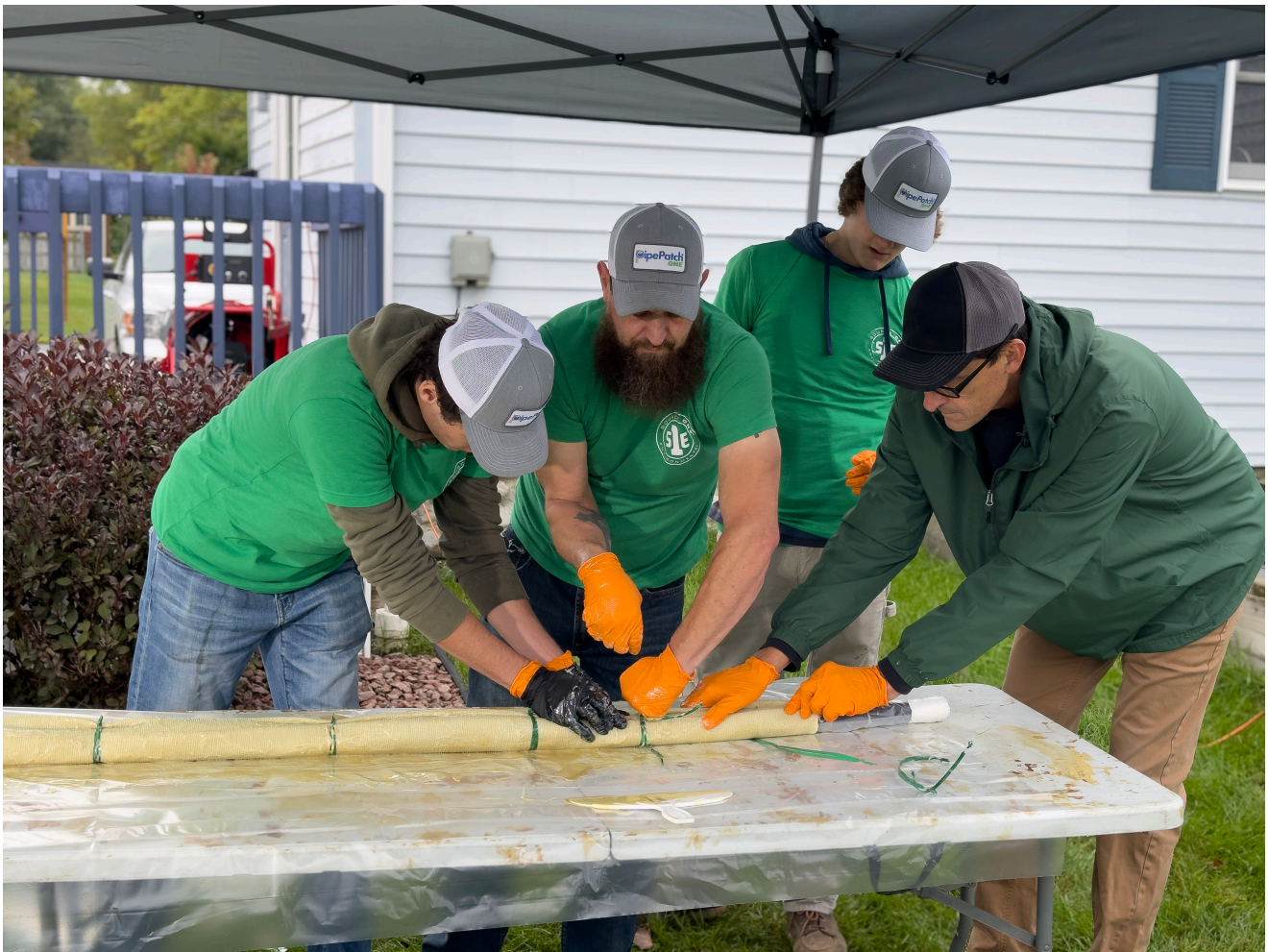
Prepping the XTEND Packer - Spot repairs offer faster solutions, targeting specific damage without the extensive downtime.
