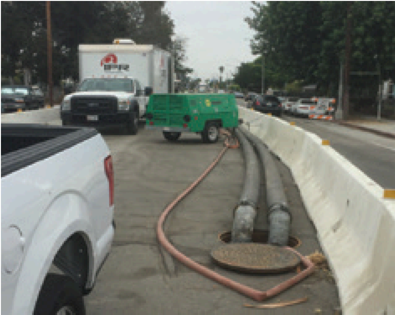
Bypass of the sewer.
