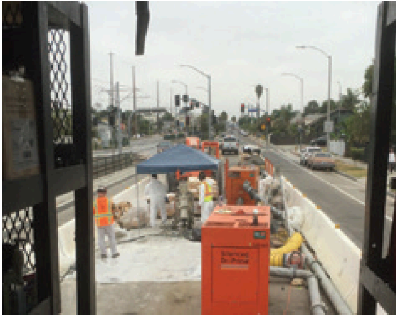
View of the construction footprint. Completed lining.
