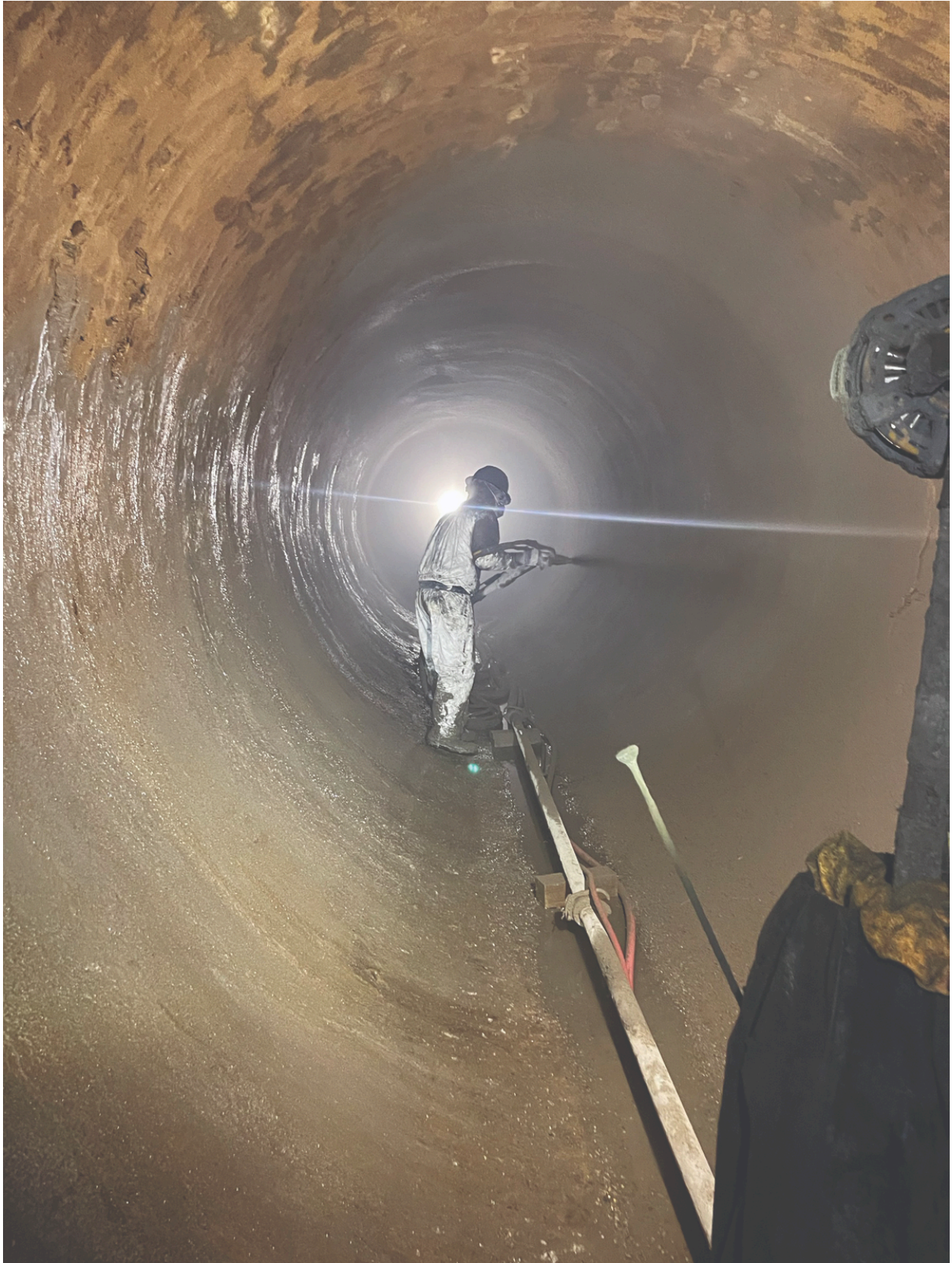
Shotcrete installation
