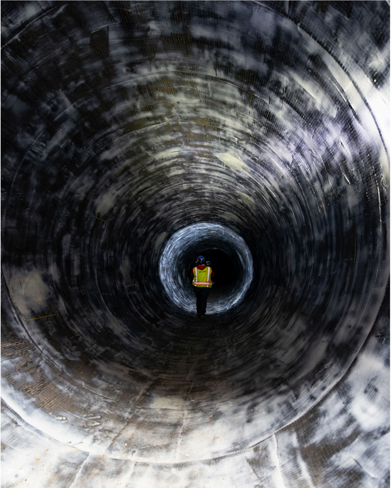
Completed CFRP installation
