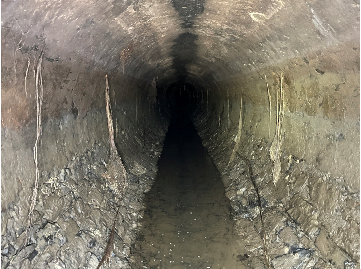
Condition of aqueduct before repairs
