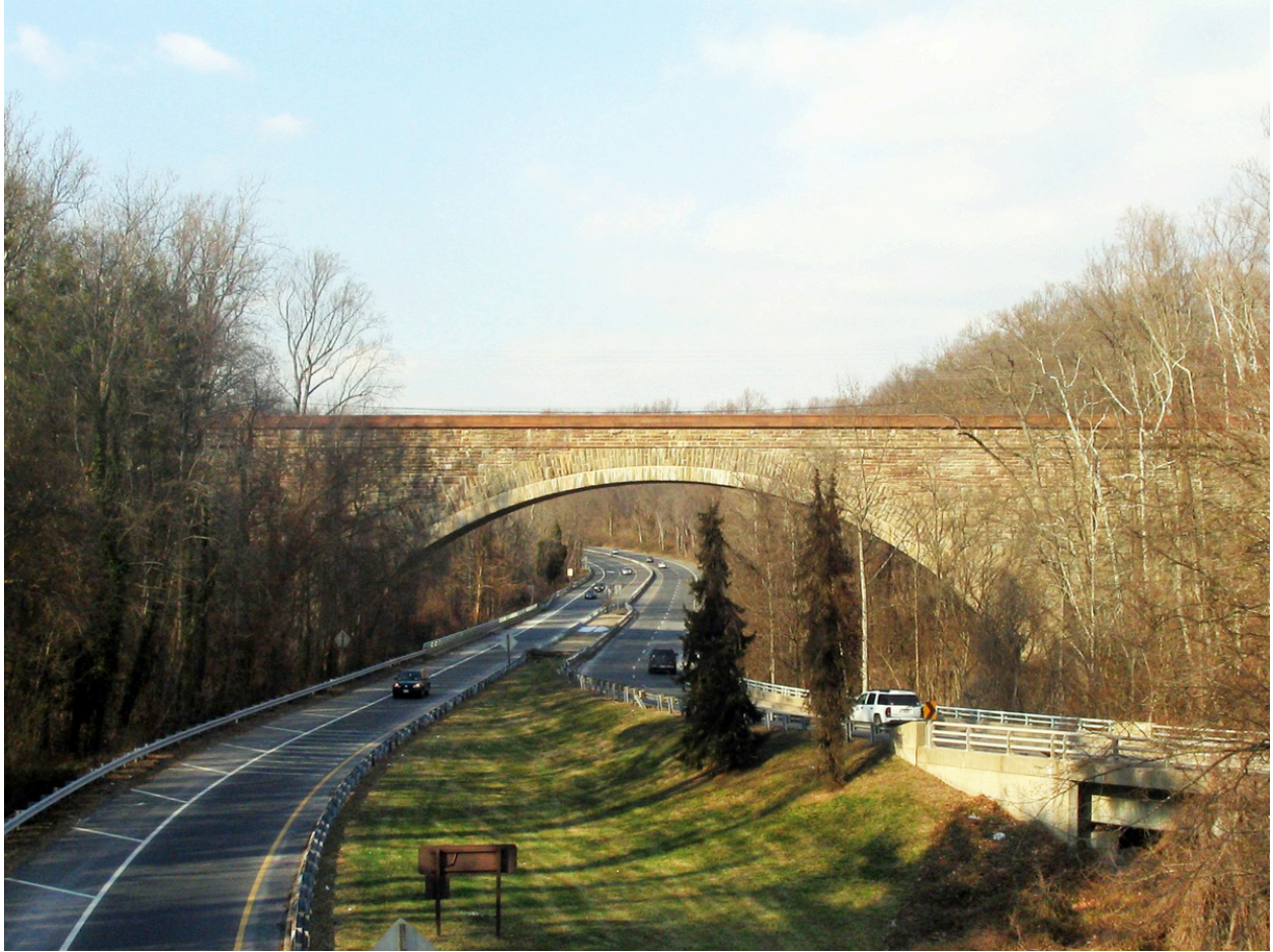
10-mile aqueduct repairs will serve community for years to come
