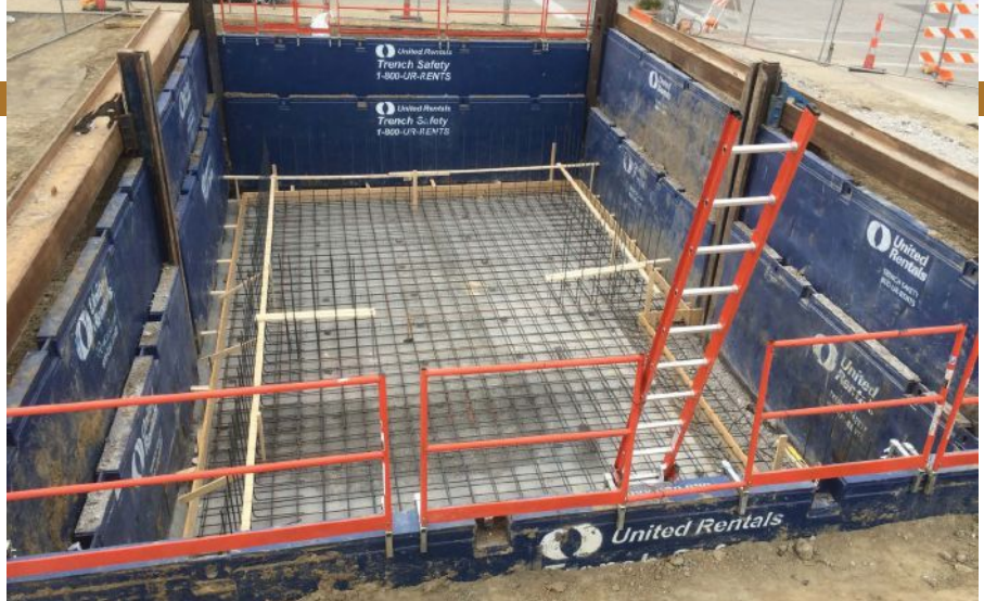
Four-sided slide rail system with tie-back beams
