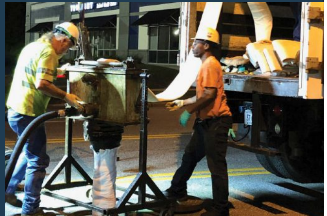
air inversion steam cured SB Liner
