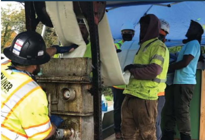
SB liner UV cure inversion liner
