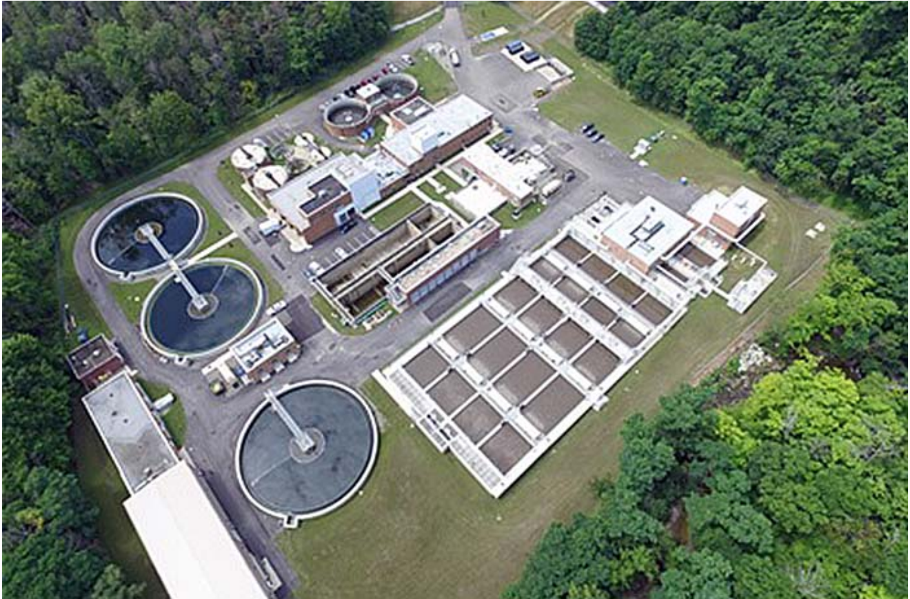
Overhead view of the North Olmsted Wastewater Treatment Plant
