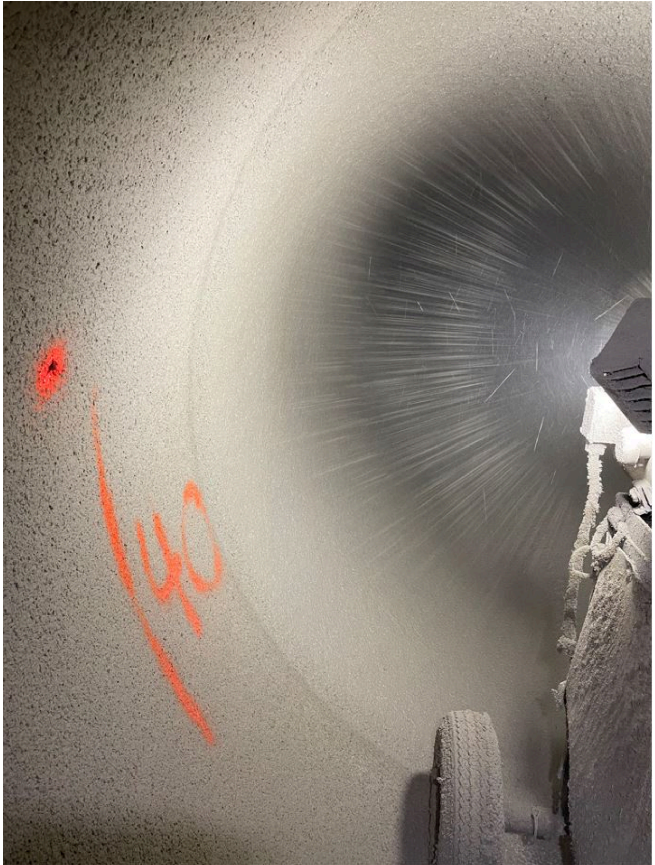
GeoSpray HCE installation via centrifugal force
