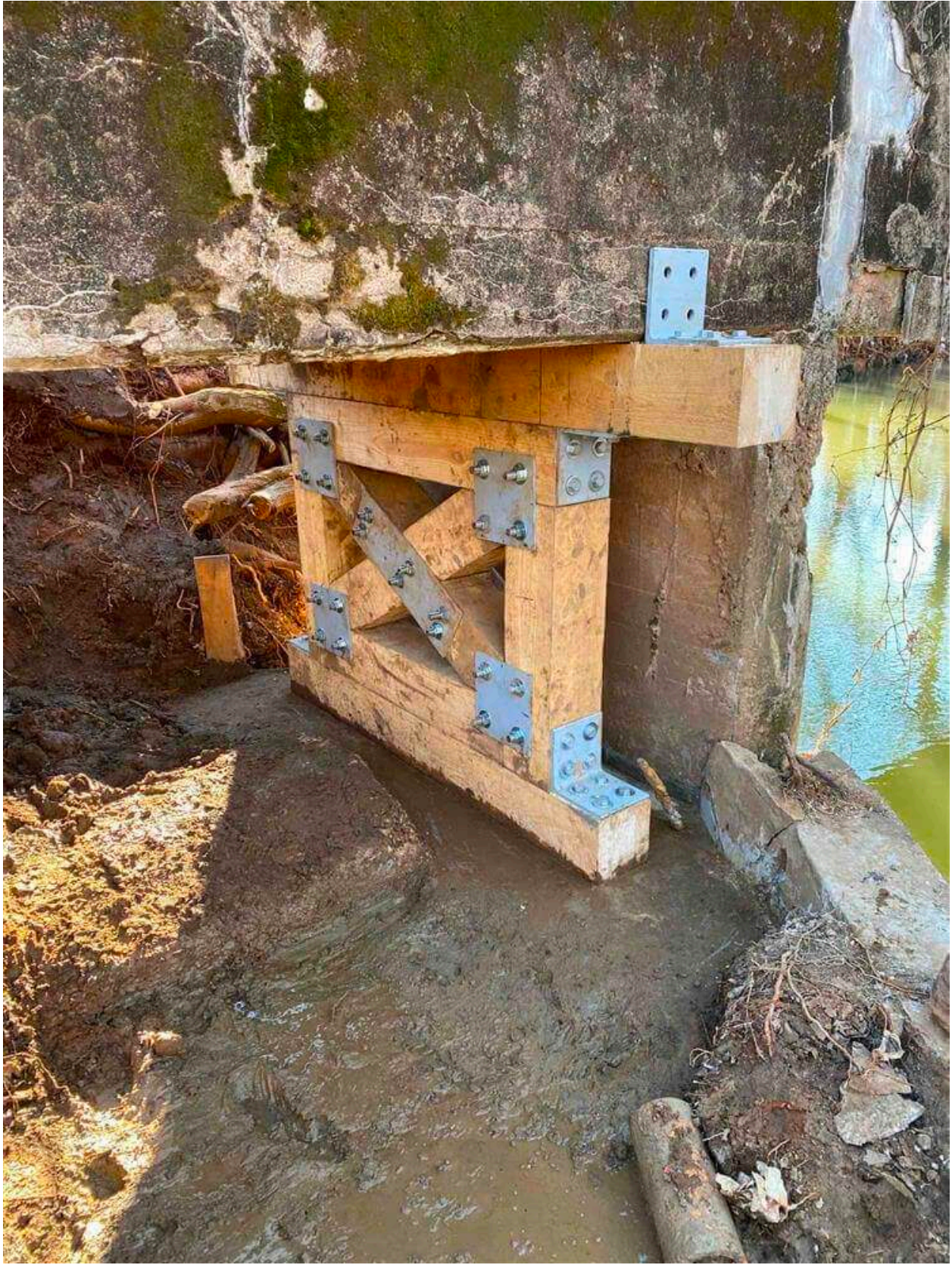
Emergency shoring was installed prior to access road construction and repairs.
