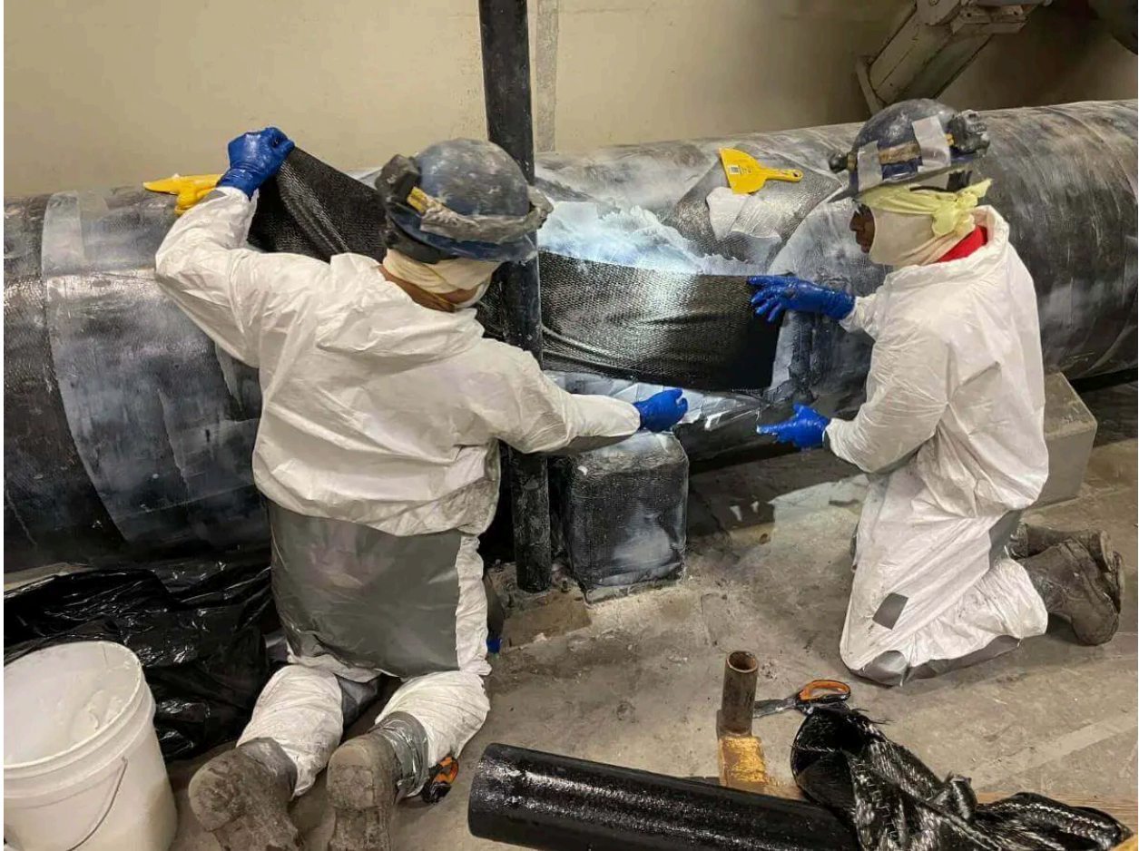
Installation of CSS V-Wrap™ Carbon Fiber system
