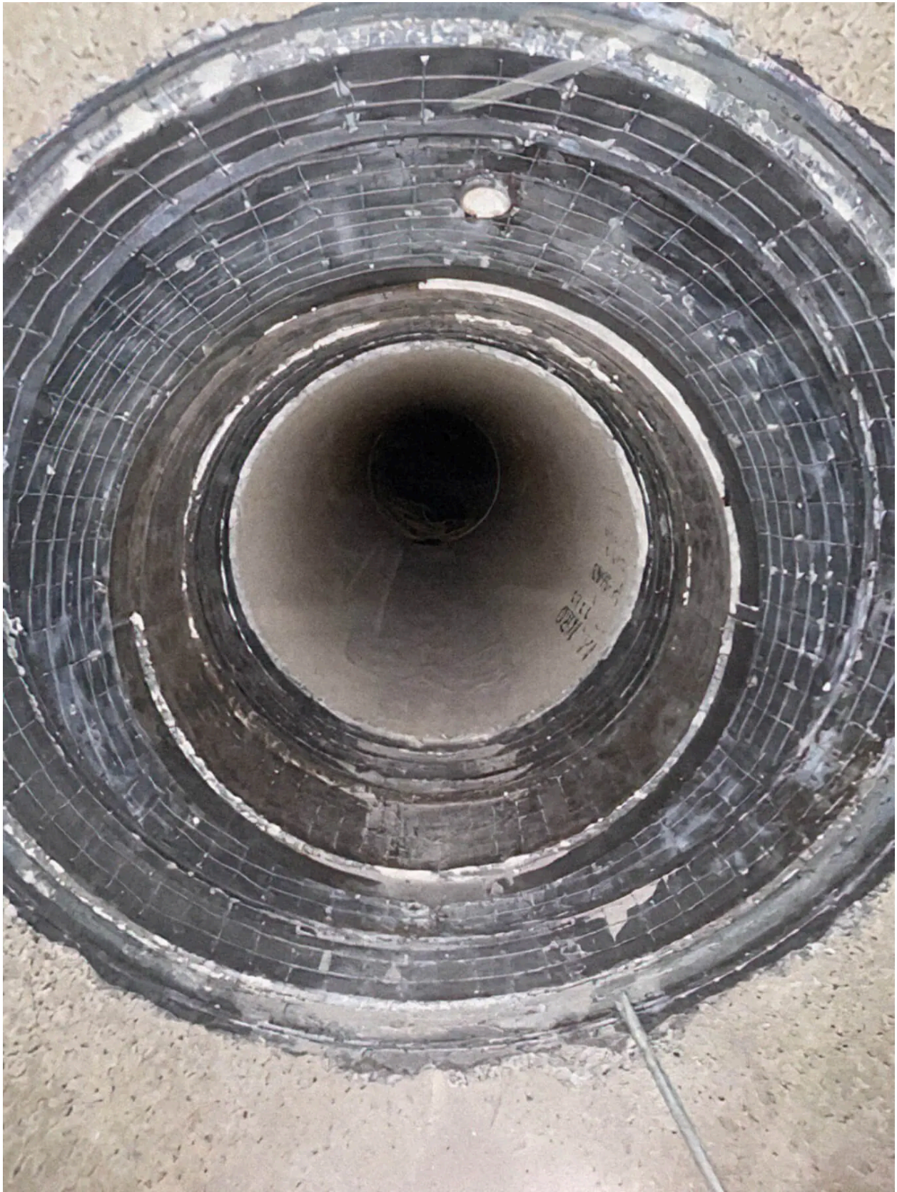
Completed restoration of pipeline
