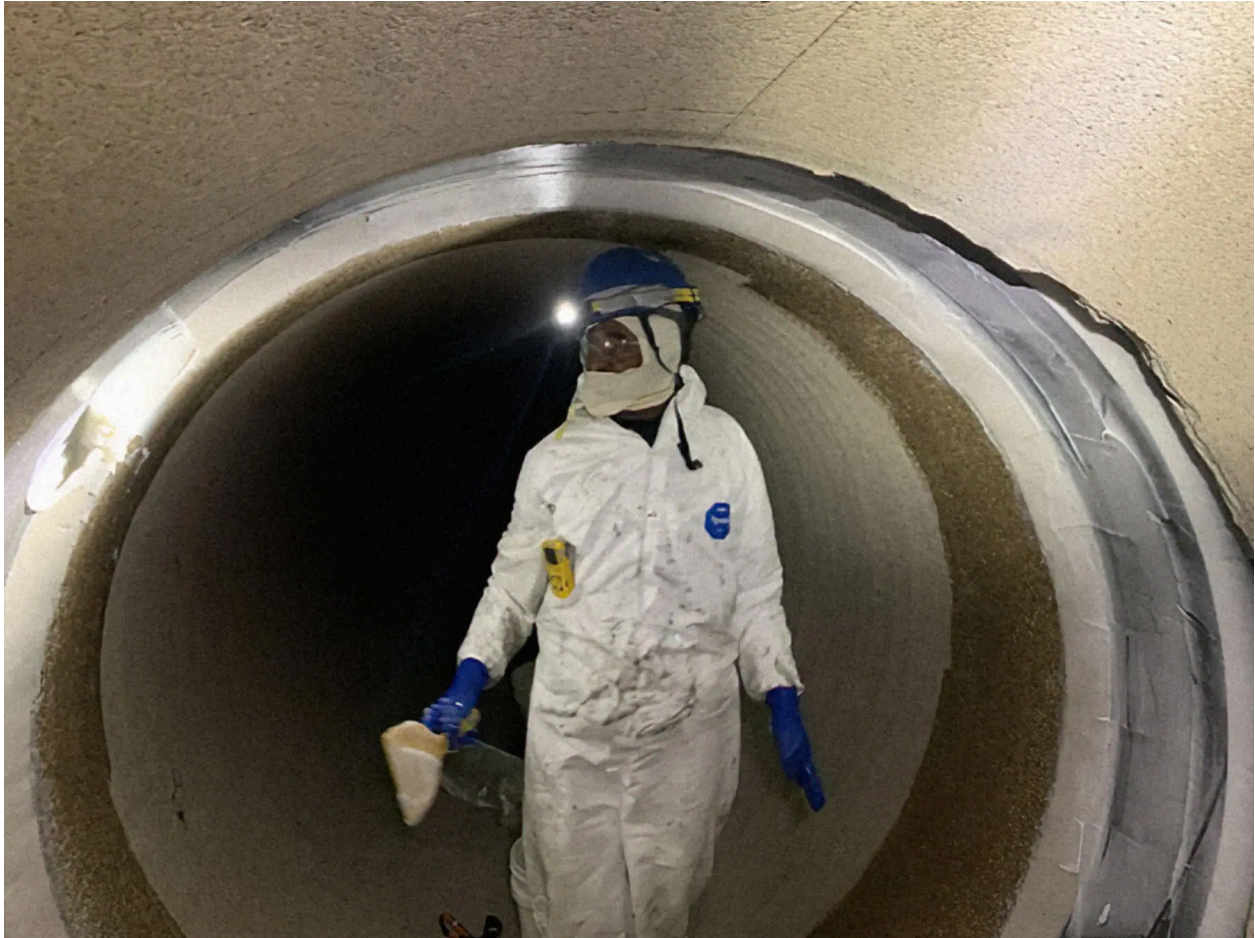
Installation of StrongPIPE® V-Wrap™ Carbon Fiber System
