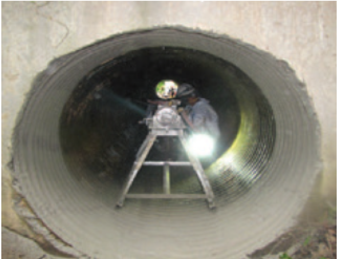
Starting of the GeoSpray Lining.
