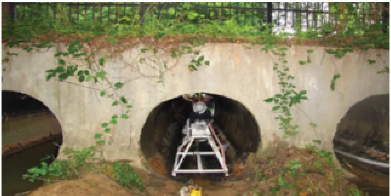
The casting equipment being positioned in the pipe prior to GeoSpray mortar application.
