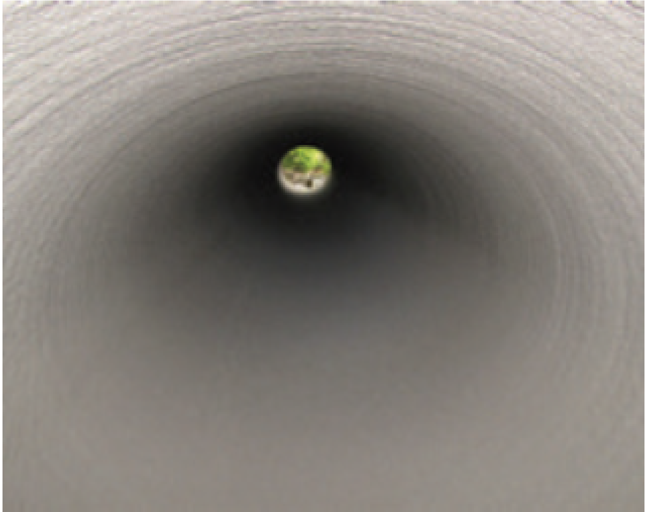
The completed 1" GeoSpray mortar lining.
