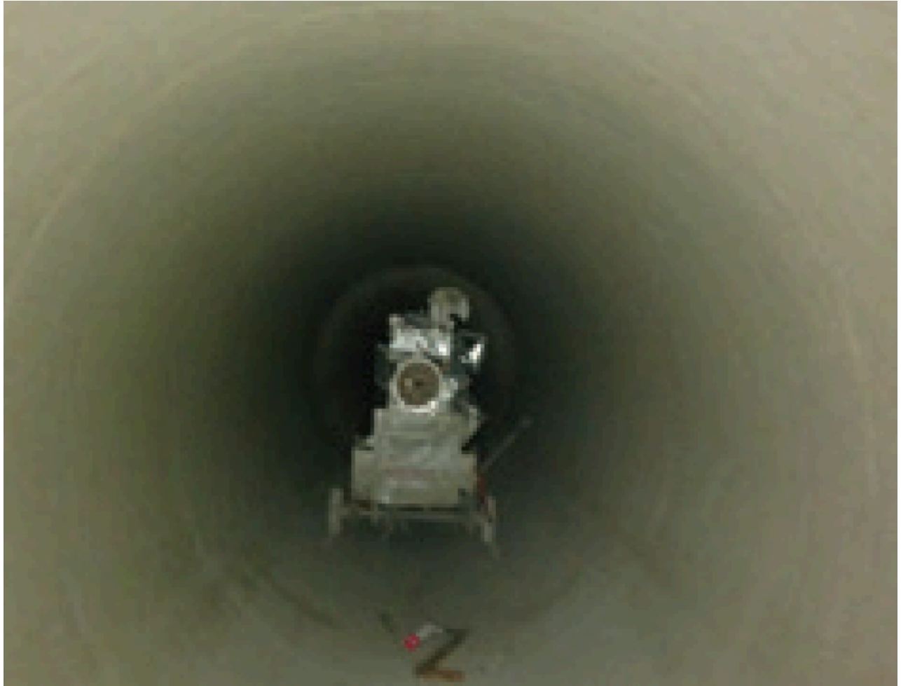
The pipe was sprayed with GeoSpray mortar to a twoinch thickness
