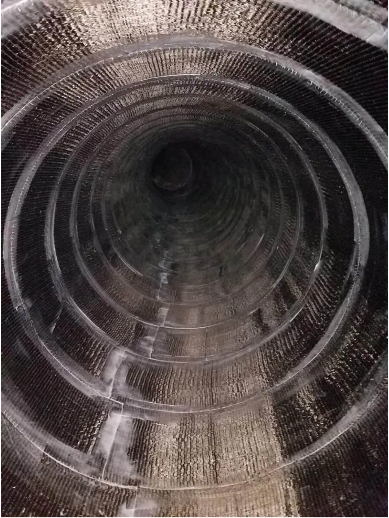
Completed renewal rotated
