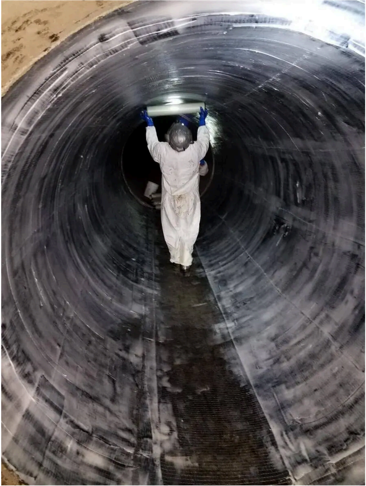
StrongPIPE®-V-Wrap™ Carbon Fiber System Installation rotated
