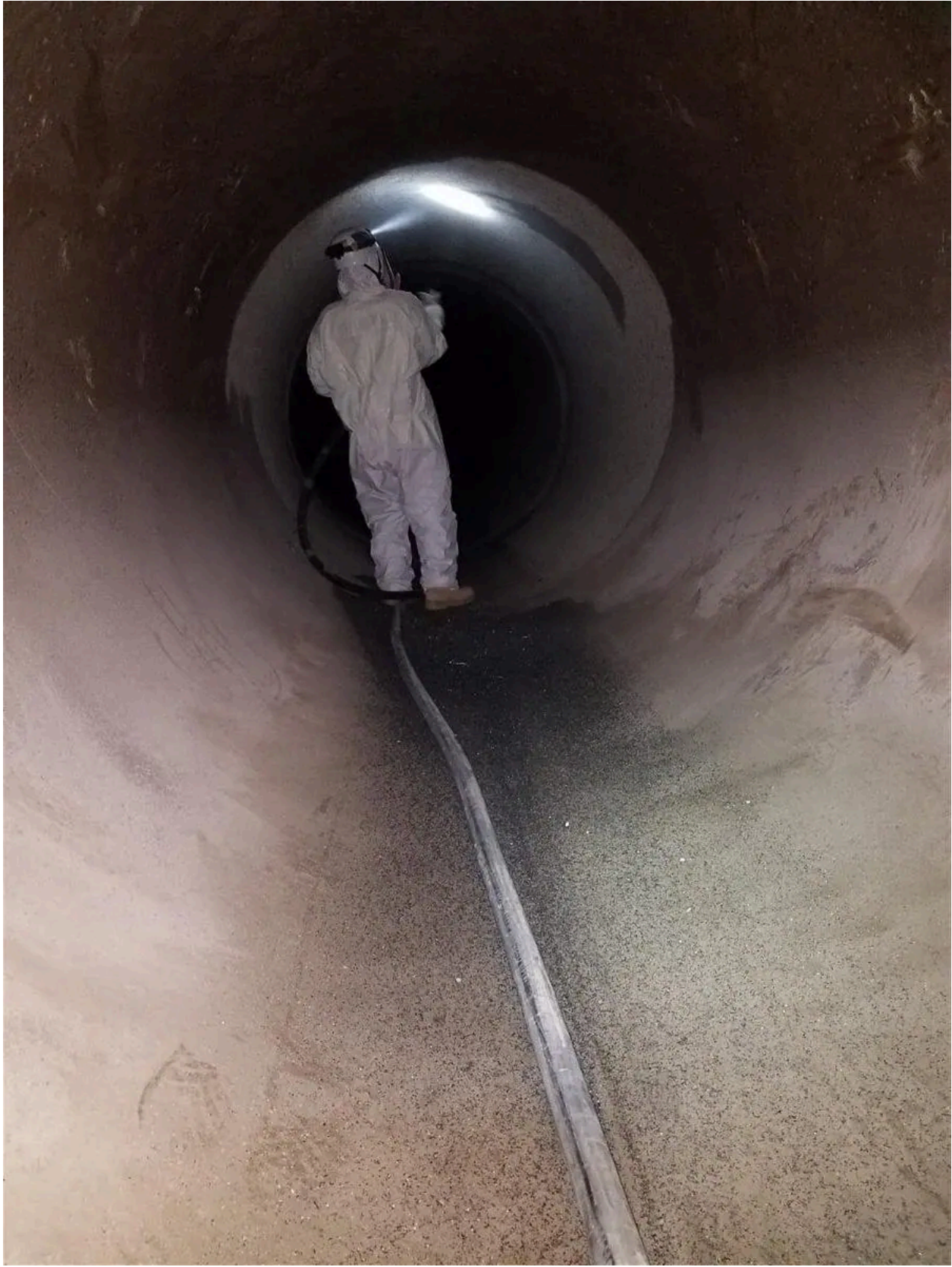
78 inch diameter pipeline required emergency renewal rotated
