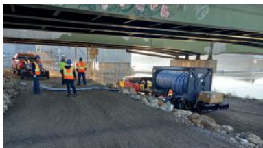
Rehabilitation of the 20-inch water line running under the Vermont Street bridge over the Kansas River.
