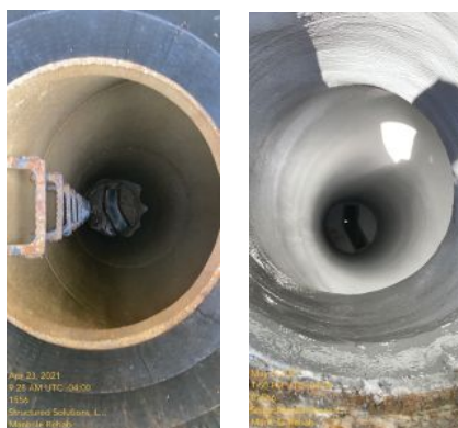
Figure 1. A manhole showing signs of corrosion and degradation (left) is restored with Dura-Plate 6000 (right) using a single-leg sprayer.
