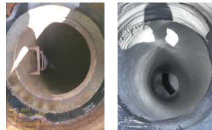
Figure 3. Steps can also be a weak point in the structure when dealing with I&I issues; removing the steps ensures a monolithic liner, eliminating weak points.
