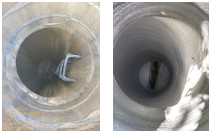
Figure 2. Corroded steps (left) are removed during restoration, which prevents workers from entering the confined space without safety equipment.
