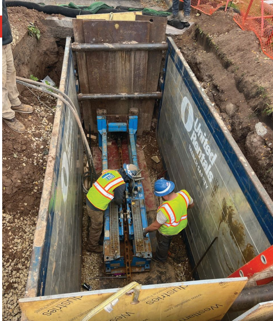
Crews utilized 10-ft trench boxes to accommodate the Grundoburst static bursting equipment.
