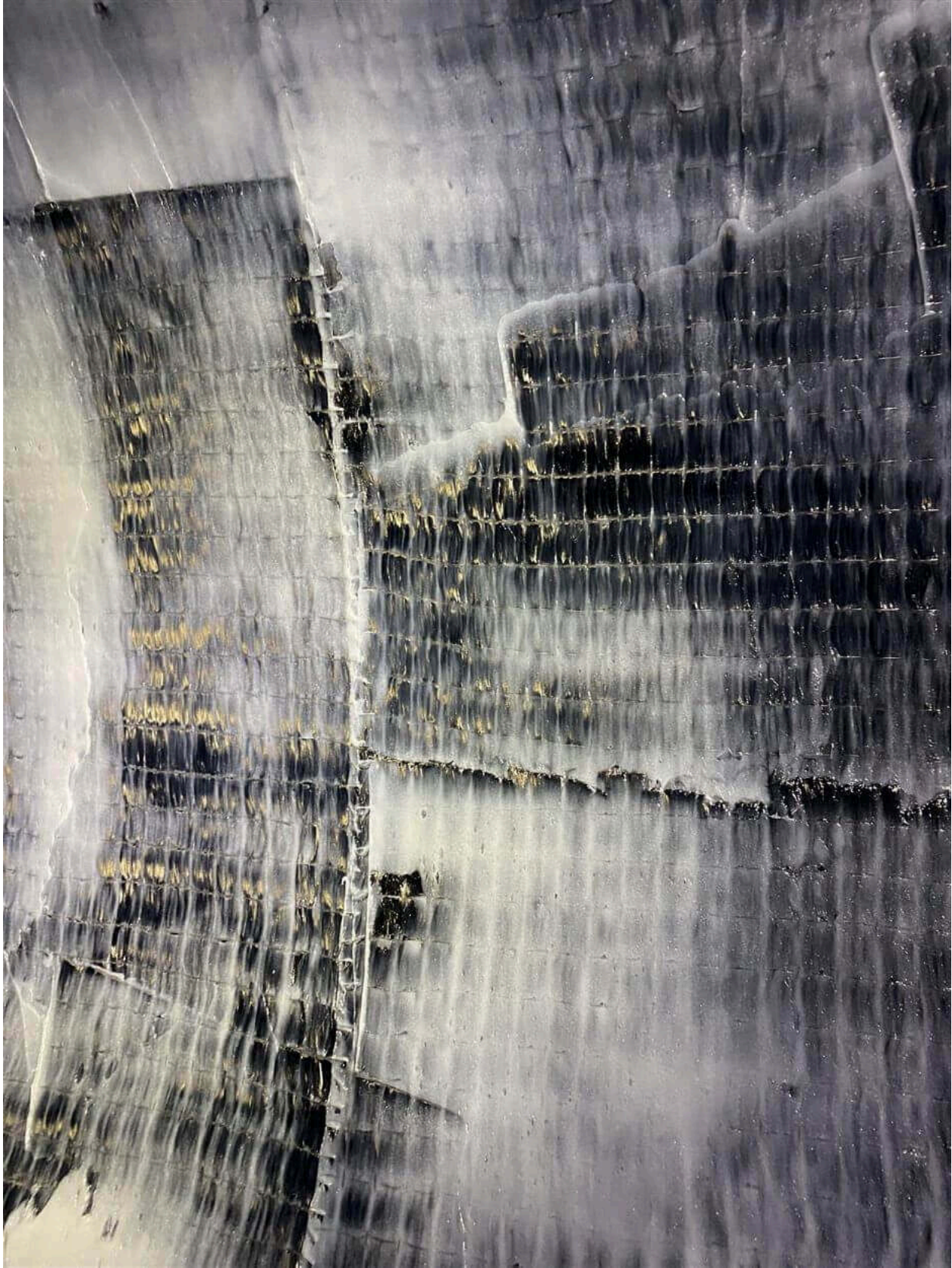
StrongPIPE® V-Wrap™ is internally applied to 16 LF of the pipeline.
