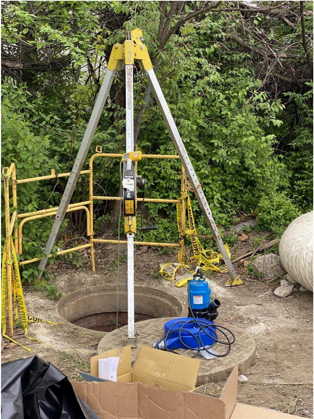
Access point to affected pipe section.
