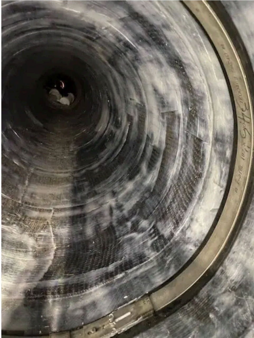
Completed StrongPIPE® V-Wrap™ installation restores the pipe's structural capacity.
