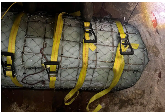
AM-Liner designed a temporary wire mesh, chain link fence and ratchet-strapped bridge to span the 10-ft wide manhole.
