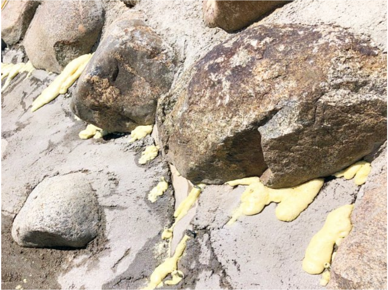
SealBoss® Seawall Repair | Cold Joint | Crack
