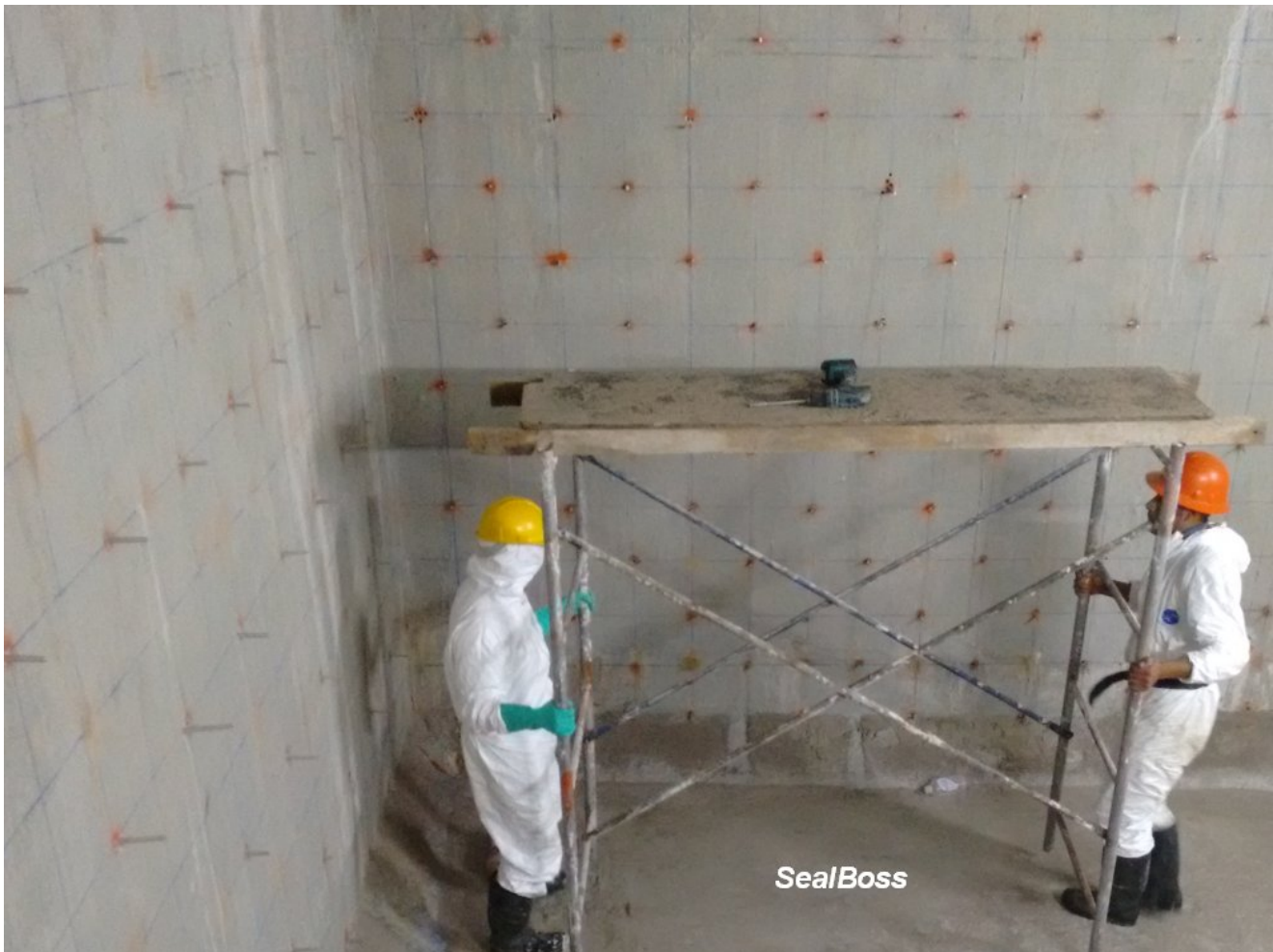
Curtain Injection Grid Pattern
