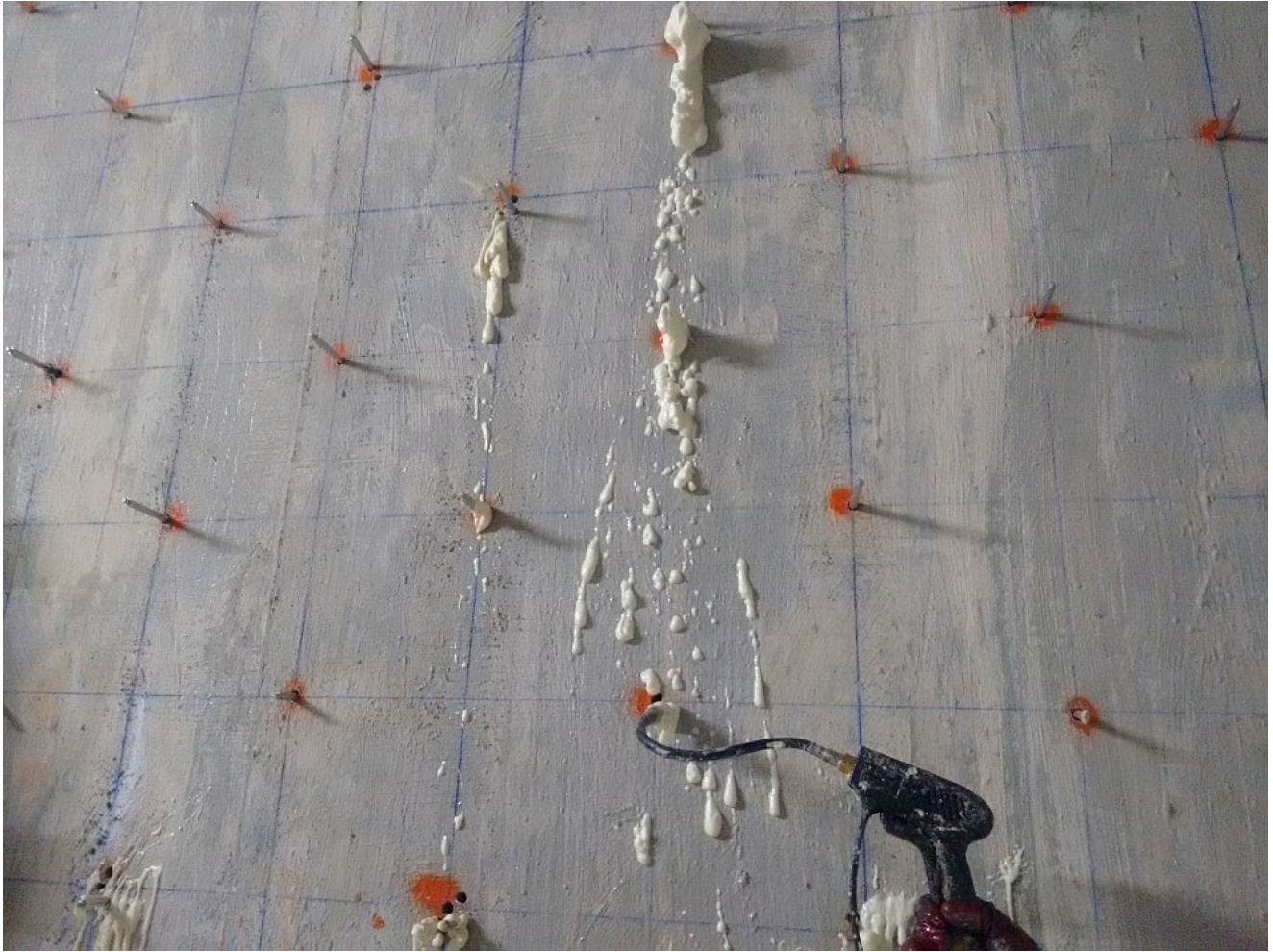
Packer Installation in a Grid Pattern
