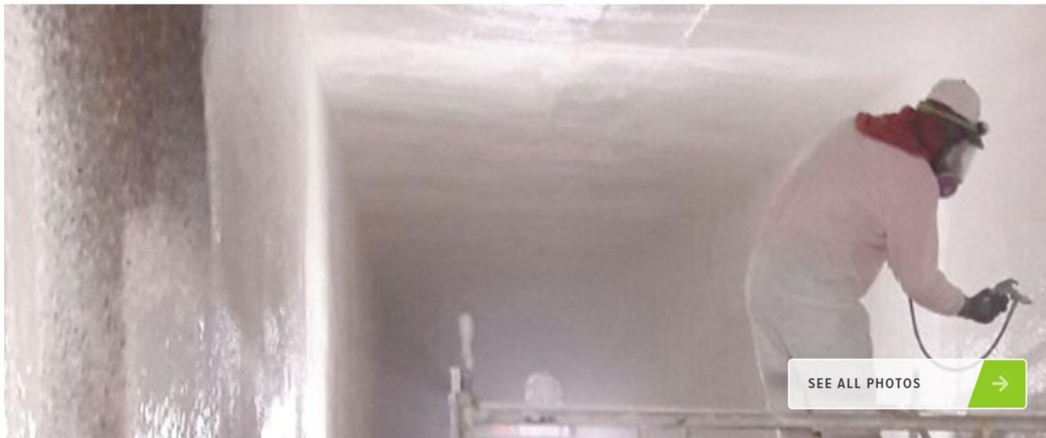
Warren Environmental's 301-14 epoxy coating system was used to protect, structurally enhance, and prevent water infiltration into the flows of the Southeast Water Pollution Control (SWPC) Plant's chlorine contact channels. Warren's epoxy coating was spray applied to the interior surfaces of 1.2 miles of 18x16 foot cast-in-place concrete channel that had suffered substantial corrosion, exposing rebar and aggregate.
