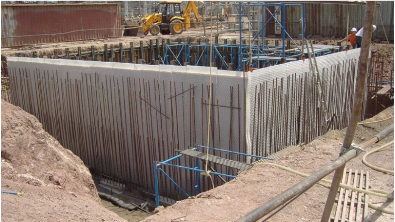
The construction site
