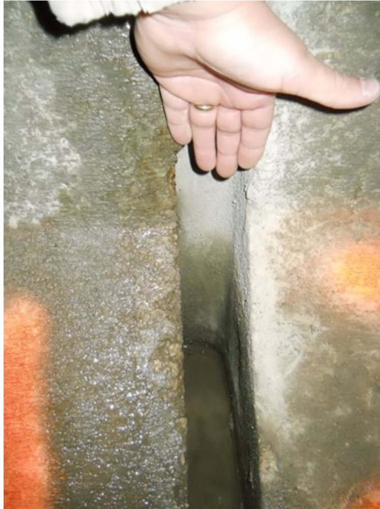
Some culvert joints were open as much as three inches.
