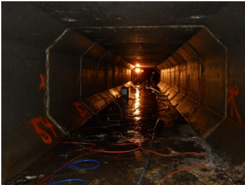
Some culvert joints were open as much as three inches.
